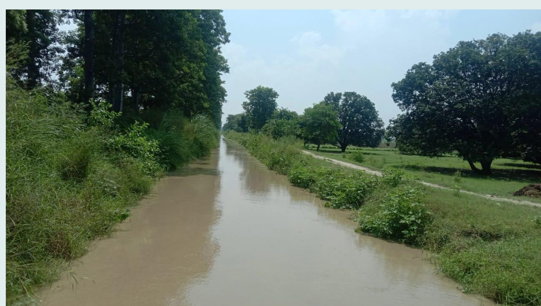
Excess Canal Water at Head Village
