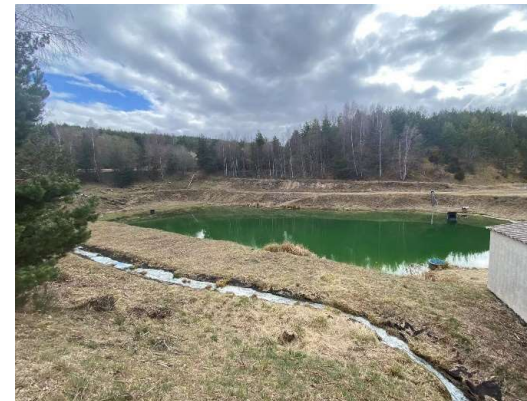
Release basin in Le Cellier
