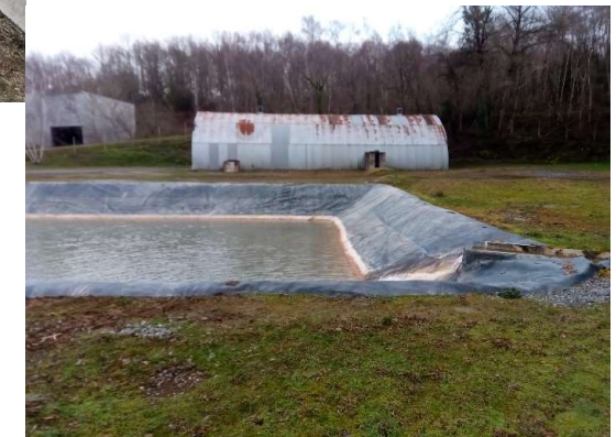
Pre-treatment basin and water treatment plan in Bellezane
