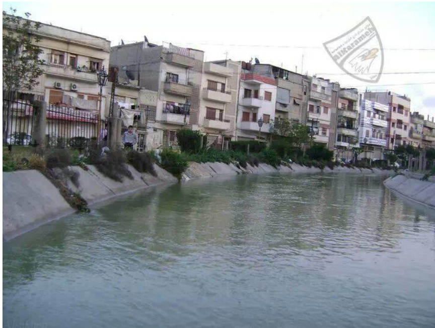
Main irrigation canal before the conflict (Homs)
