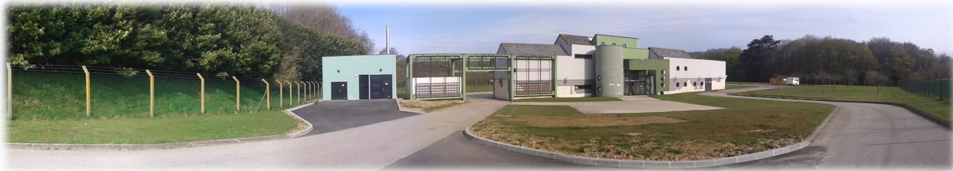
Yport drinking water station
