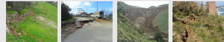
Figure 4. case and examples of landslides in great Kabylia: a), b) Azazga, c) Illiltén, d) Tizgirt
