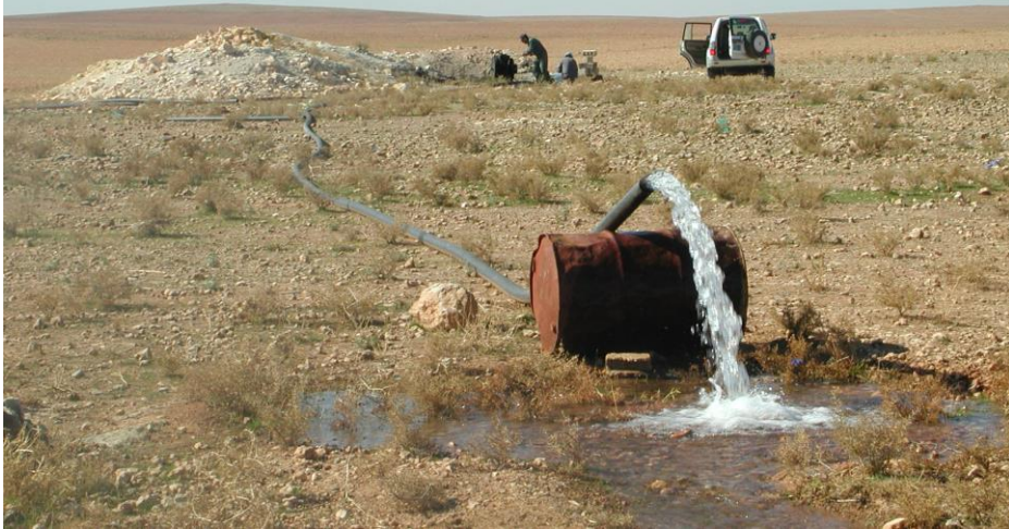
Pumping test of a new well in the Salamiah region
