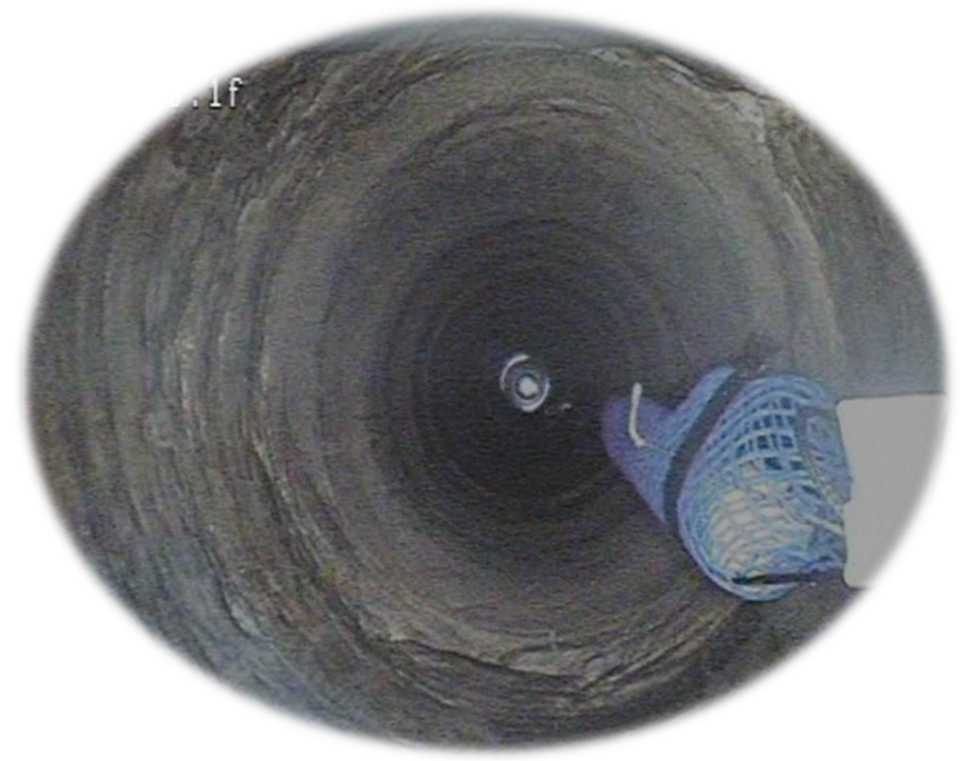
Video Confirmation of Depth and Alignment with respect to Target Fracture Prior to Liner Installation
