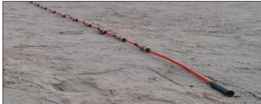
Electrode string installed into the piezometre
